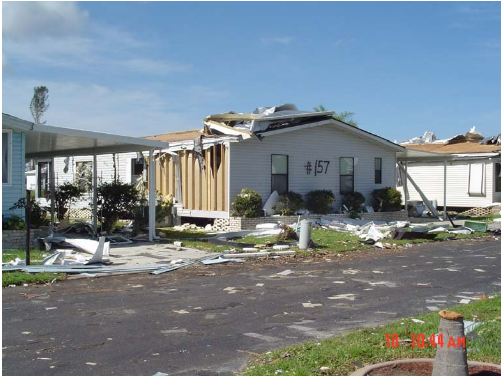
Figure 4-18. Examples of Carports on Leeward Side of Manufactured Homes Faring Relatively Well (note extensive structure damage on windward side).
