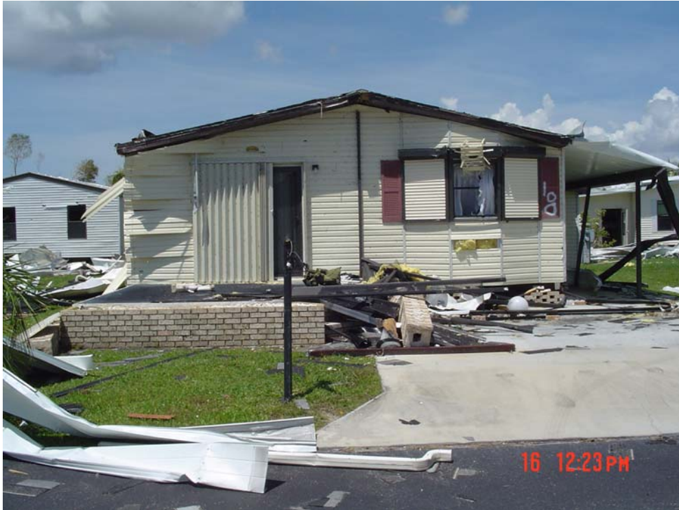
Figure 4-20. Example of Patio Enclosure and Carport Collapse Along Front of Home with Carport Section on Side of Home Still Standing.
