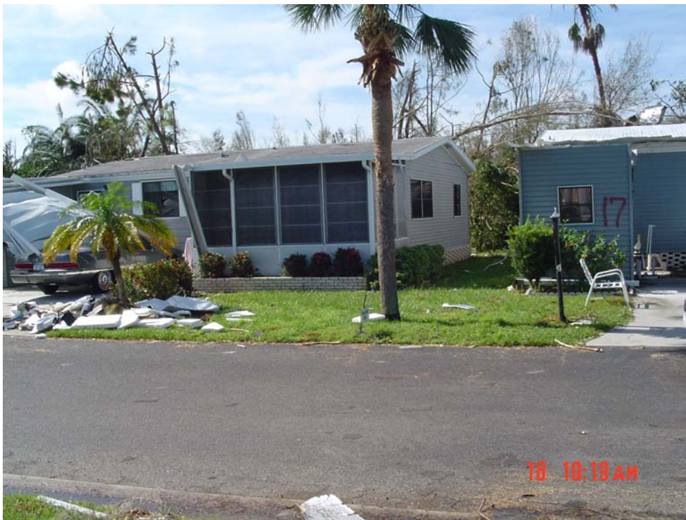
Figure 4-19. Example of Solid-Walled Patio Enclosure that Fared Well (note complete collapse of adjoining carport).
