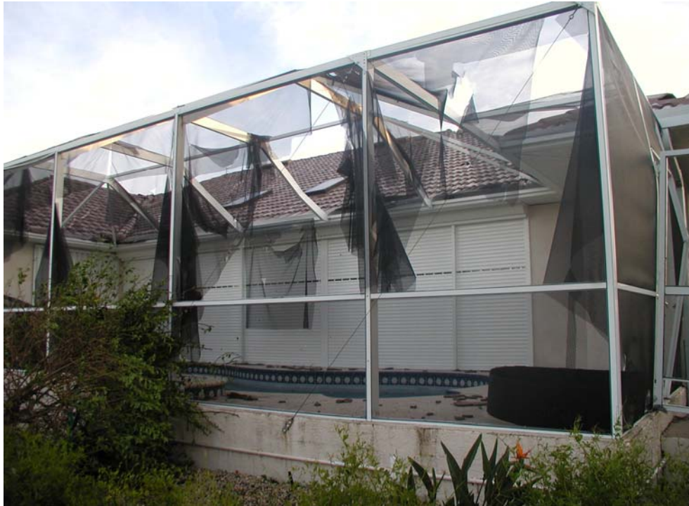
Figure 4-2. Example of a Partially Failed Aluminum Screen Enclosure.
